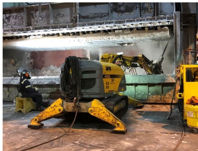
Figure 7. Brokk 400 at work in a 115-tonne furnace (author's image).
