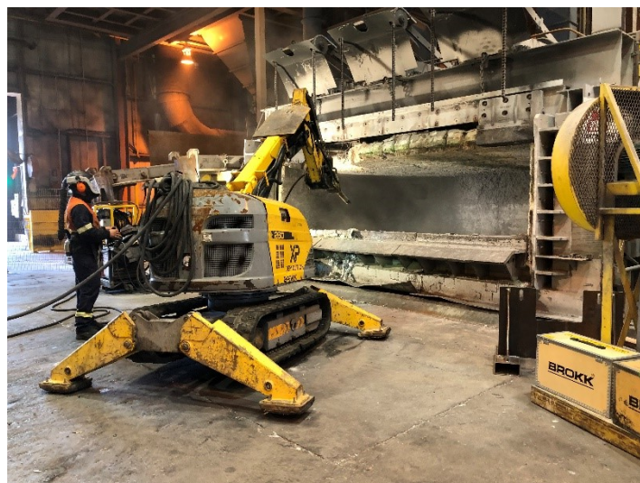
Figure 11. Operator standing close to a Brokk robot (author’s image).
