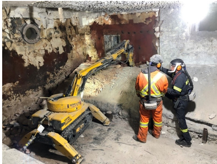
Figure 6. One of the first trials with a small Brokk unit in 2020 (author's image).
