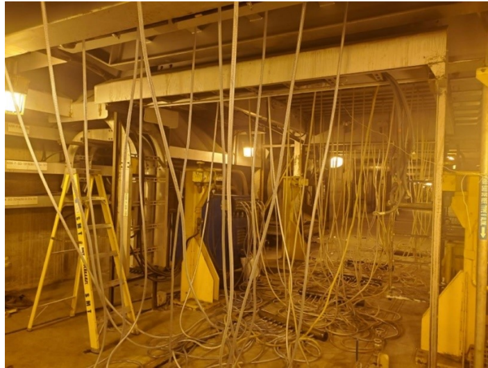
Figure 10. Vacuum hoses and manifolds used during the full-scale trial (author’s image).
